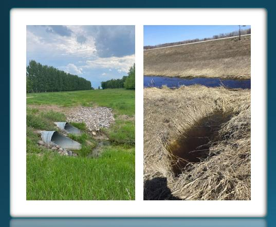
RLWD hired Anderson Excavating to fix a small washout created by over land flooding off a hay field.
